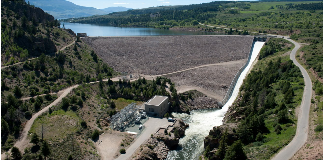
Figure 1.—A summer release through the spillway at Green Mountain Dam and Reservoir. Green Mountain Powerplant, located just below the dam, also generates power.
